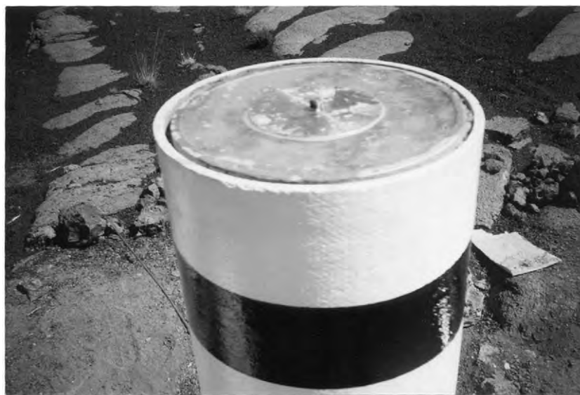
Fig. 6. Detail of a monument of the Fogo Geodetic Network. Forced centring is achieved with a WILD thread on a steel plate imbedded in cement. The inner concrete pipe is filled with reinforced concrete with a 1-m 3 foundation, and is separated from the outer pipe by fibreglass for thermal insulation (Berberan, 1997). Special care was taken to select geologically stable sites to build the monuments.
