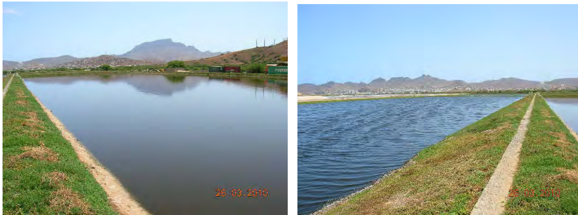
Fig. 1-2. Basins at the sewage plant, São Vicente, 26 March 2010 (Cornelis J. Hazevoet)
